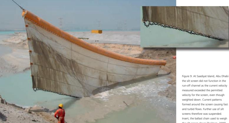
measured exceeded the permitted velocity for the screen, even though weighted down. Current patterns formed around the screen causing fast and turbid flows. Further use of silt screens therefore was suspended. Insert, the ballast chain used to weigh the silt screen down (Taelman, 2009).
