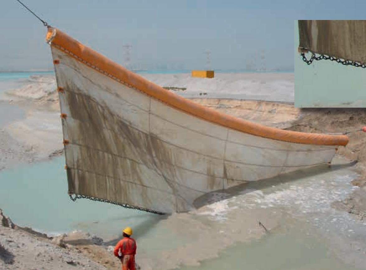
Figure 9. At Saadiyat Island, Abu Dhabi the silt screen did not function in the run-off channel as the current velocity measured exceeded the permitted velocity for the screen, even though weighted down. Current patterns formed around the screen causing fast and turbid flows. Further use of silt screens therefore was suspended. Insert, the ballast chain used to weigh the silt screen down (Taelman, 2009).
