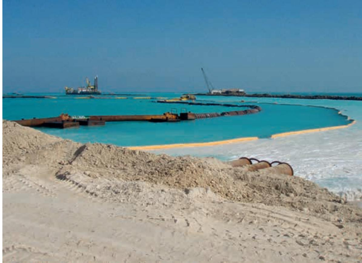
Figure 10. A hanging silt screen at a dredging project in the Arabian Gulf at a reclamation discharge was applied successfully in combination with a breakwater and minimal current velocity.
