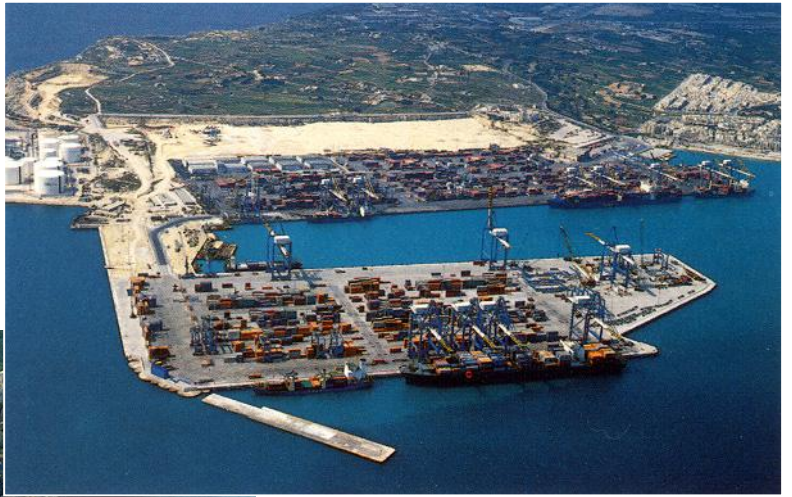
Realised new port, 1999
