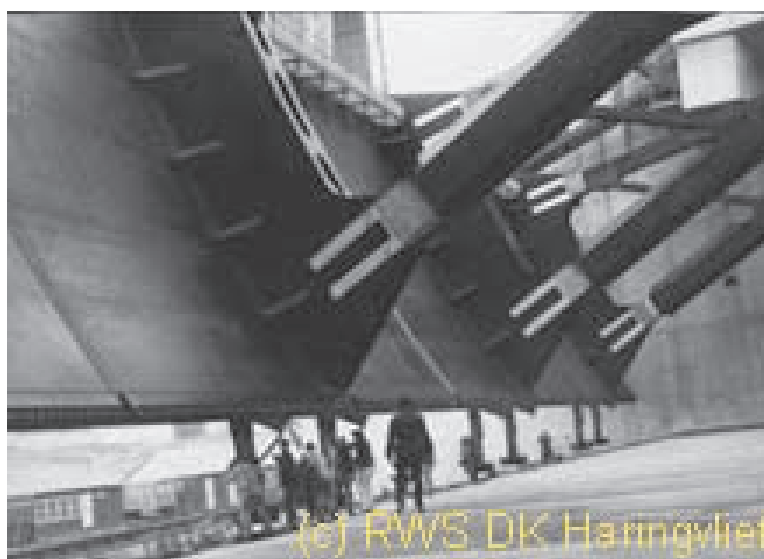
Figure 5.22: Haringvliet barrier during construction.
