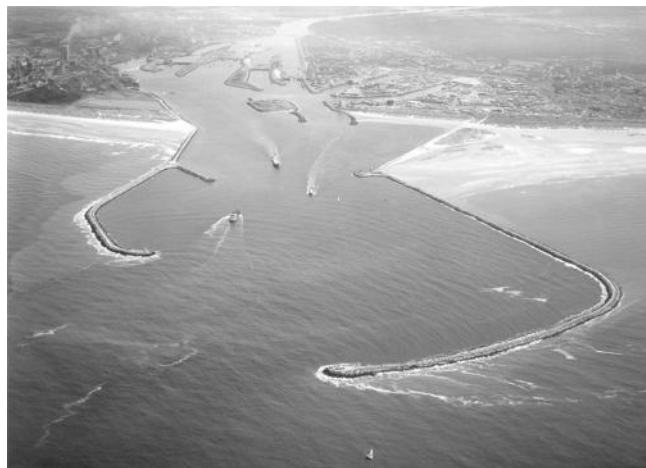
Figure 1.1: The breakwater at the harbour of IJmuiden, The Netherlands. One can clearly see the influence of the breakwater on the wave propagation. (CIRIA et al., 2007)
